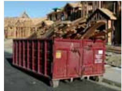
Figure 3 Disposal or delivery? This is wood waste paid for 3 times: purchase, site handling (several times), and disposal.
