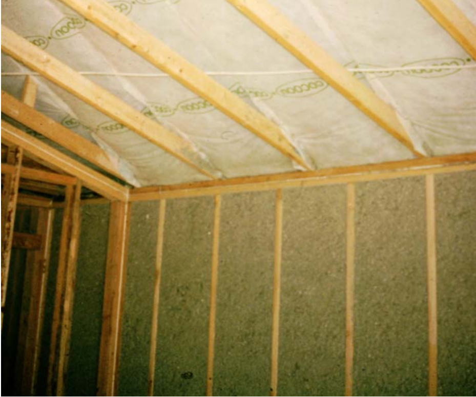
Photograph 3: Netted Cellulose – Air and vapour permeable insulation in hot-dry climate
