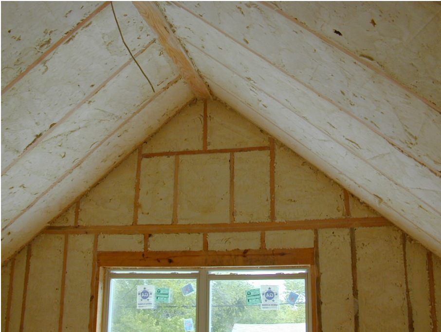
Photograph 2: Spray Foam Insulation
