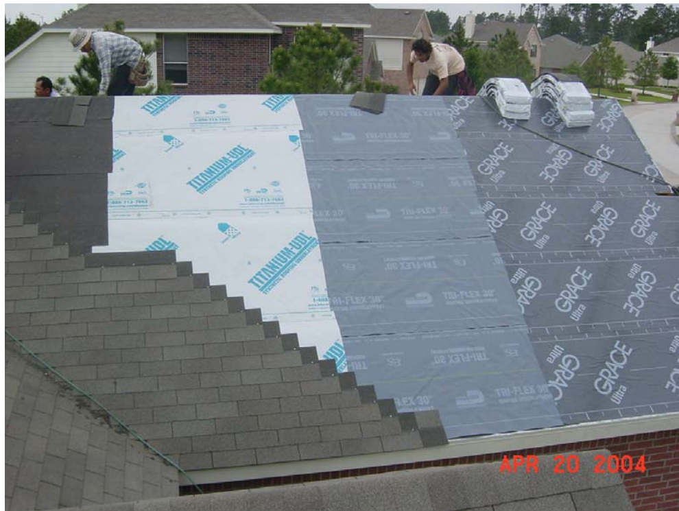
Photograph 6: Inward Moisture Drive Experiment – Various permeabilities of roofing underlayment were evaluated.
